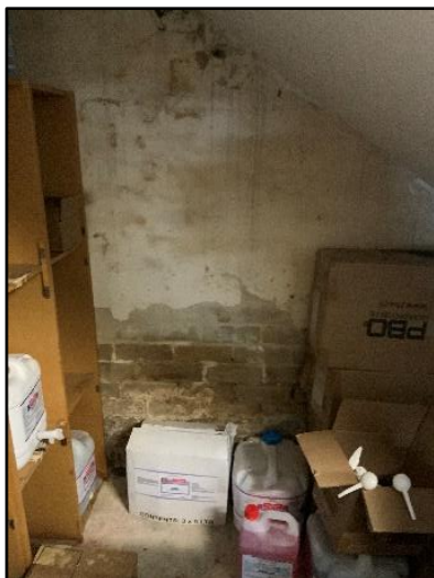
Figure 63. Internal view to storage space, basement. Note poor condition of masonry wall.
