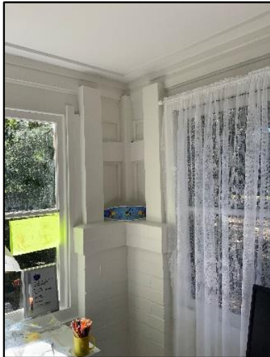
Figure 152. Internal view to brick piers of verandah in enclosed area.
