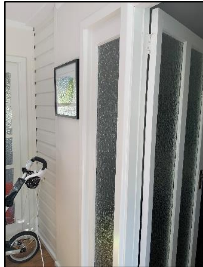
Figure 153. Internal view to weatherboard cladding of exteriors of dwelling visible in enclosed verandah space.
